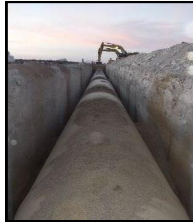
Installation of 108-inch pipe along IPL Section 17
