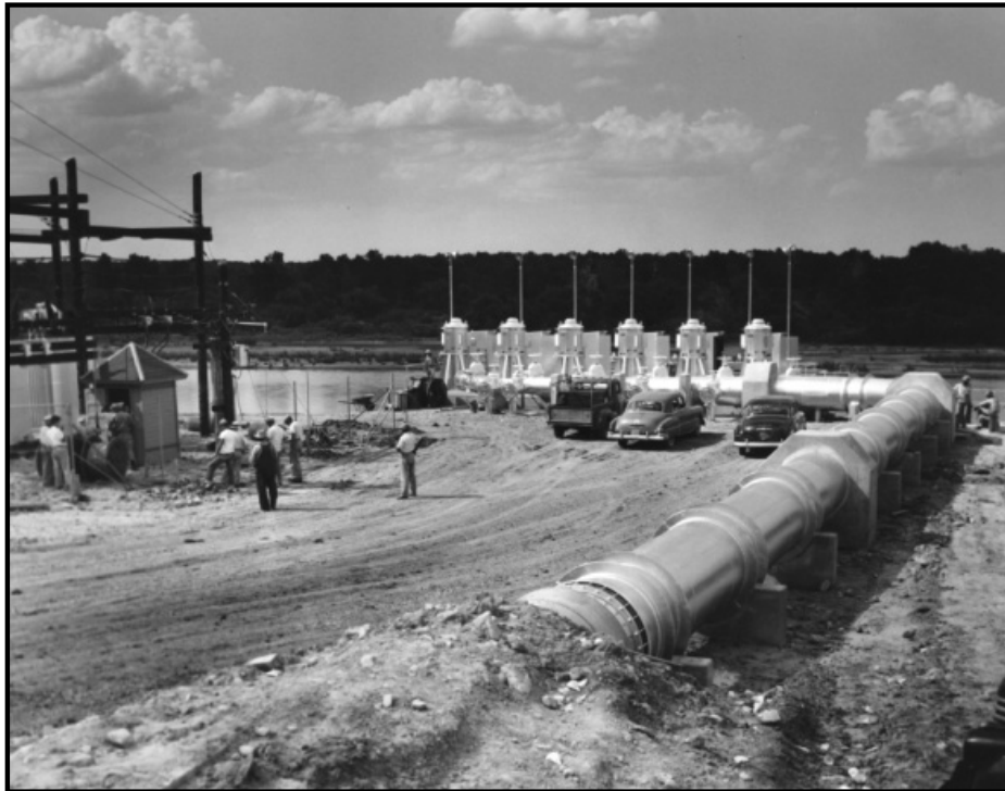
City of Dallas Red River Pump Station, 1953-1957
