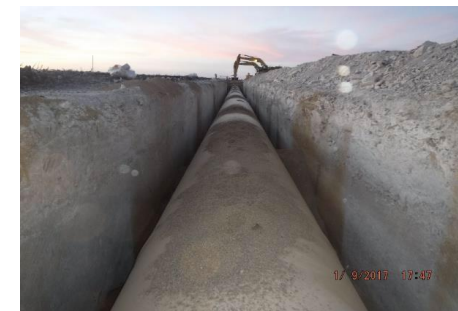
Installation of 108-inch pipe along Section 17
