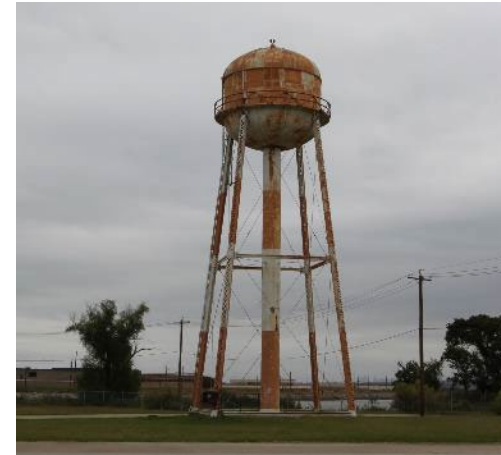
DNAS Water Tower, c. 1941
