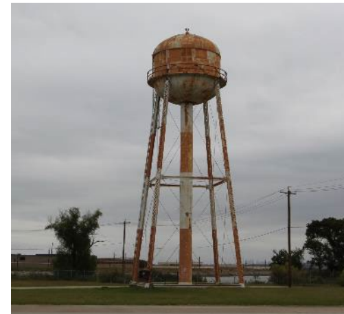
DNAS Water Tower, c. 1941
