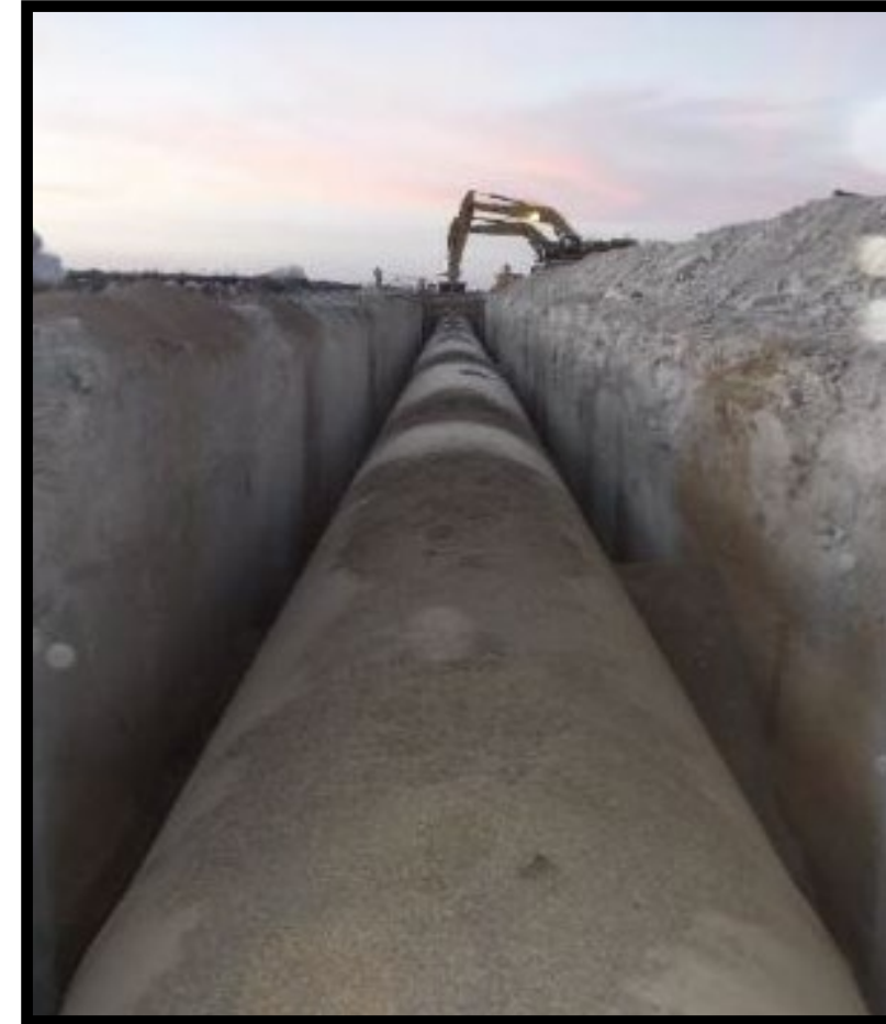
Installation of 108-inch pipe along IPL Section 17
