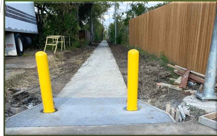
After Alley to Trail Conversion View from Edgewood St. entrance
