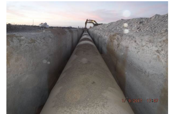
Installation of 108-inch pipe along Section 17
