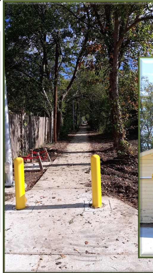
After Alley to Trail Conversion View from Jeffries St. entrance
