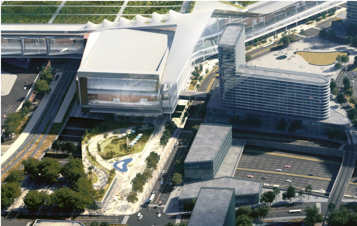
Deck Park Connects Pedestrians over I-30
