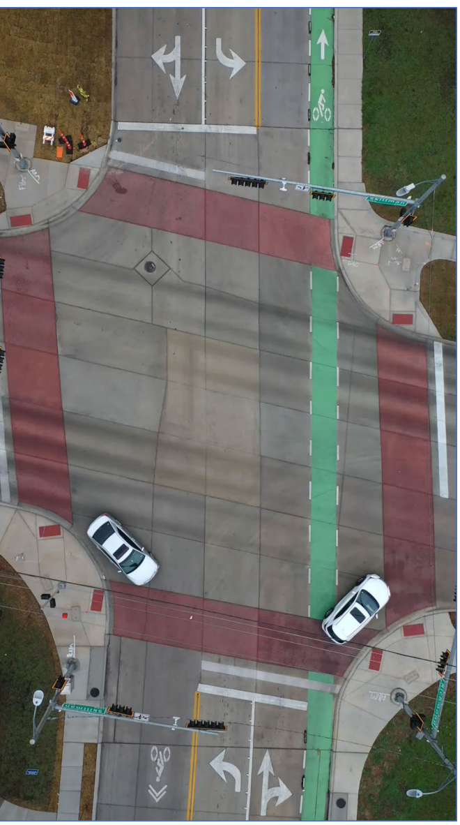
Richmond Ave at Skillman St – Post Construction Time Lapse Drone Video
