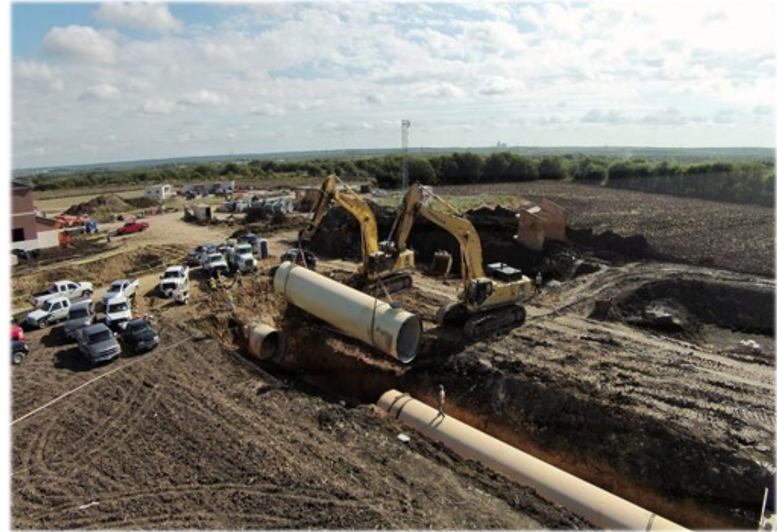
TRWD/ DWU Integrated Pipeline Project
