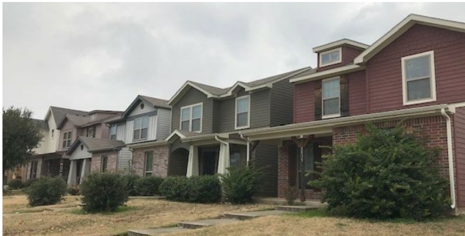
Fair Park Estates single-family homes built by Southfair Community Development Corporation
