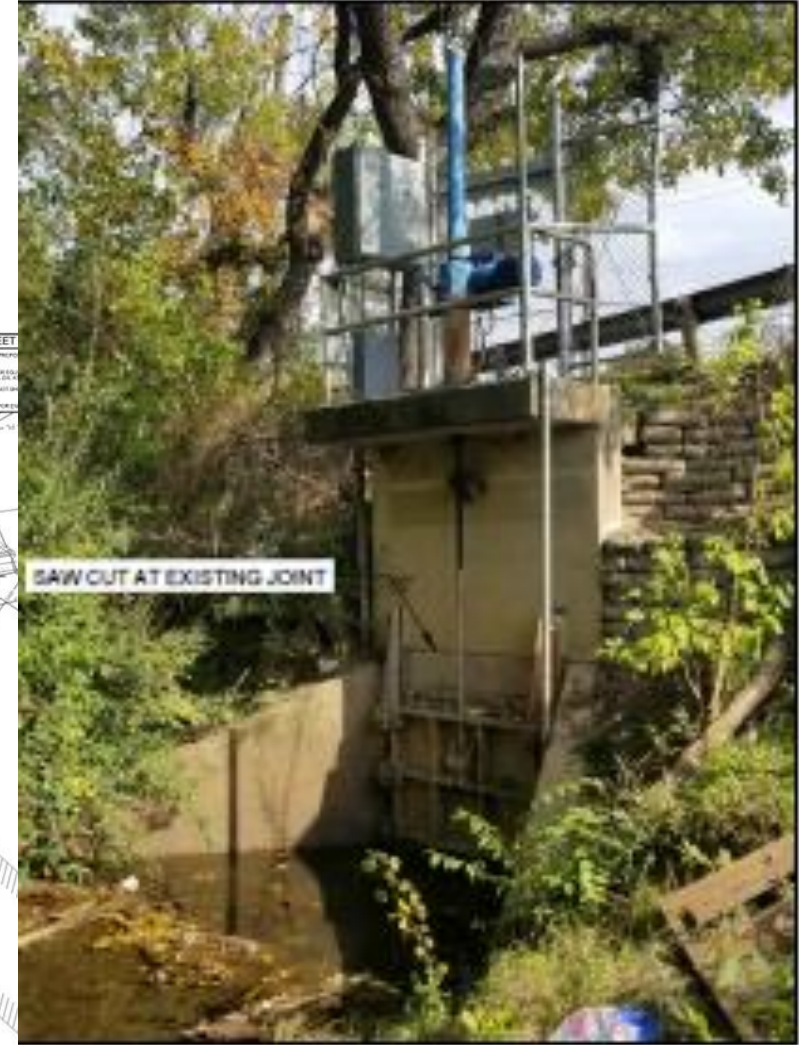
Existing Headwall & Slide Gate structure to be improved
