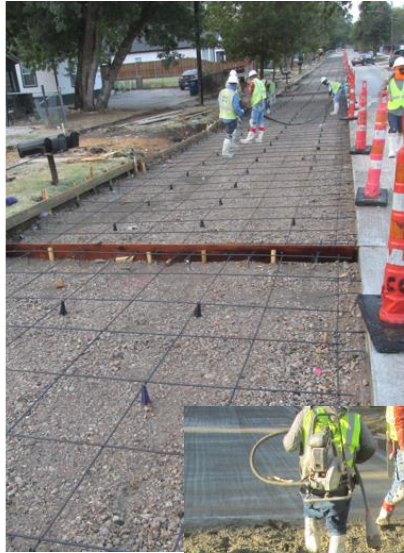
Steel Reinforced Concrete
