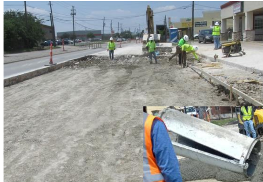
Fiber Reinforced Concrete Construction (Day 0)
