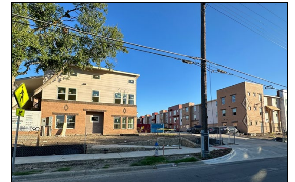
Kiva East construction is almost complete 10/2/2023
