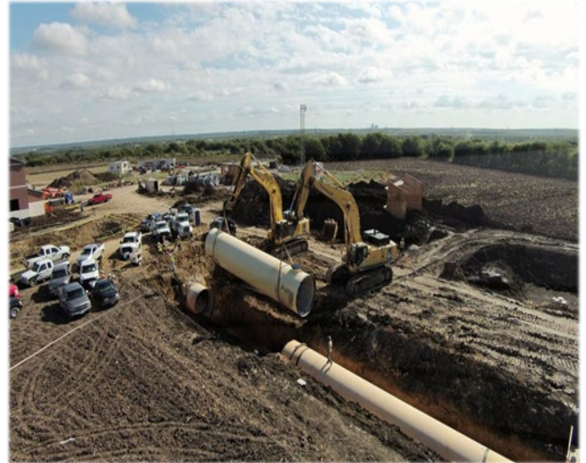
TRWD/ DWU Integrated Pipeline Project
