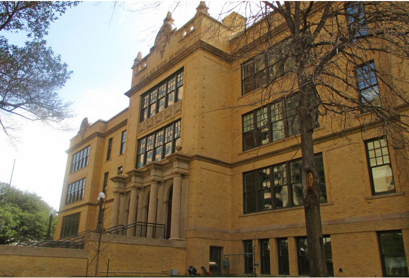
Built in 1907, Dallas High School was a public secondary school until its closing in 1995. The classical revival structure was renovated into a mixed-use property in 2017 and is a core part of the Downtown City Center District.
