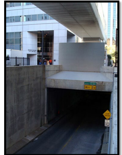
Bullington Truck Terminal
