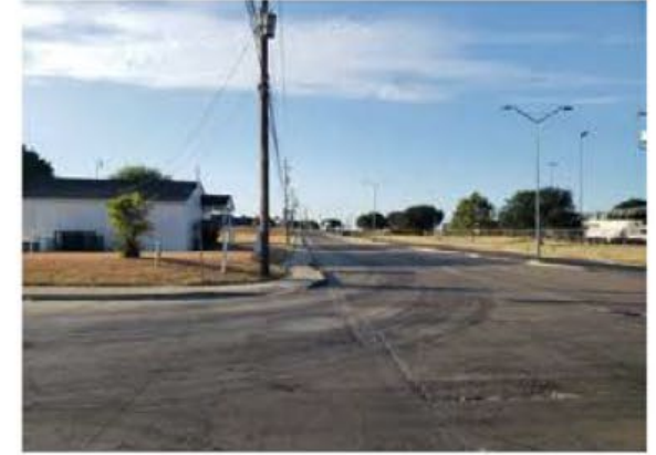
SOUTH ALONG BONNIE VIEW ROAD FROM SEC
